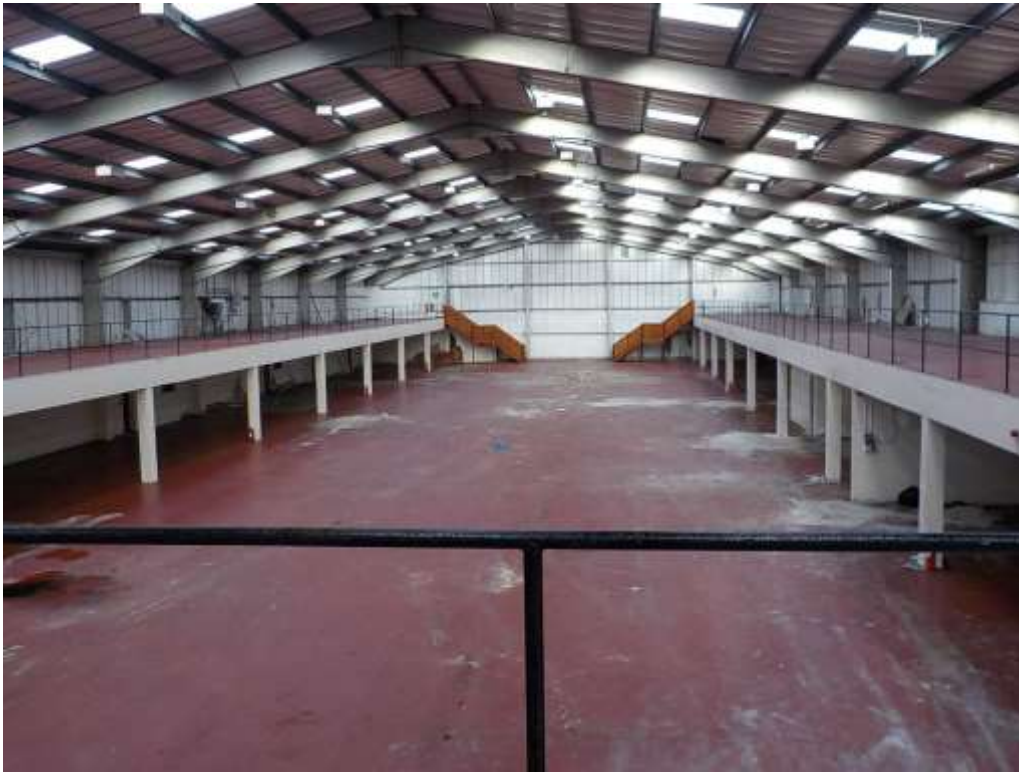
Interior of the former Blakemore Cash & Carry building
