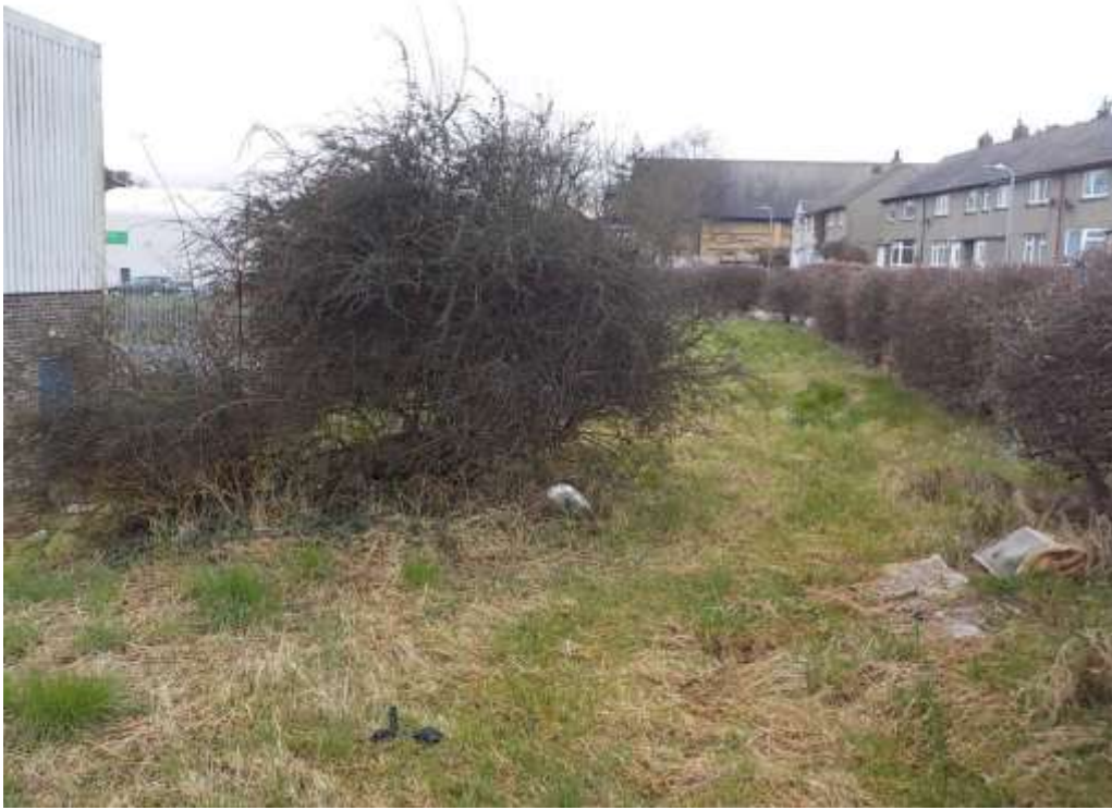
Grass bank to the rear of the building with occasional tree/shrub and hedgerow
